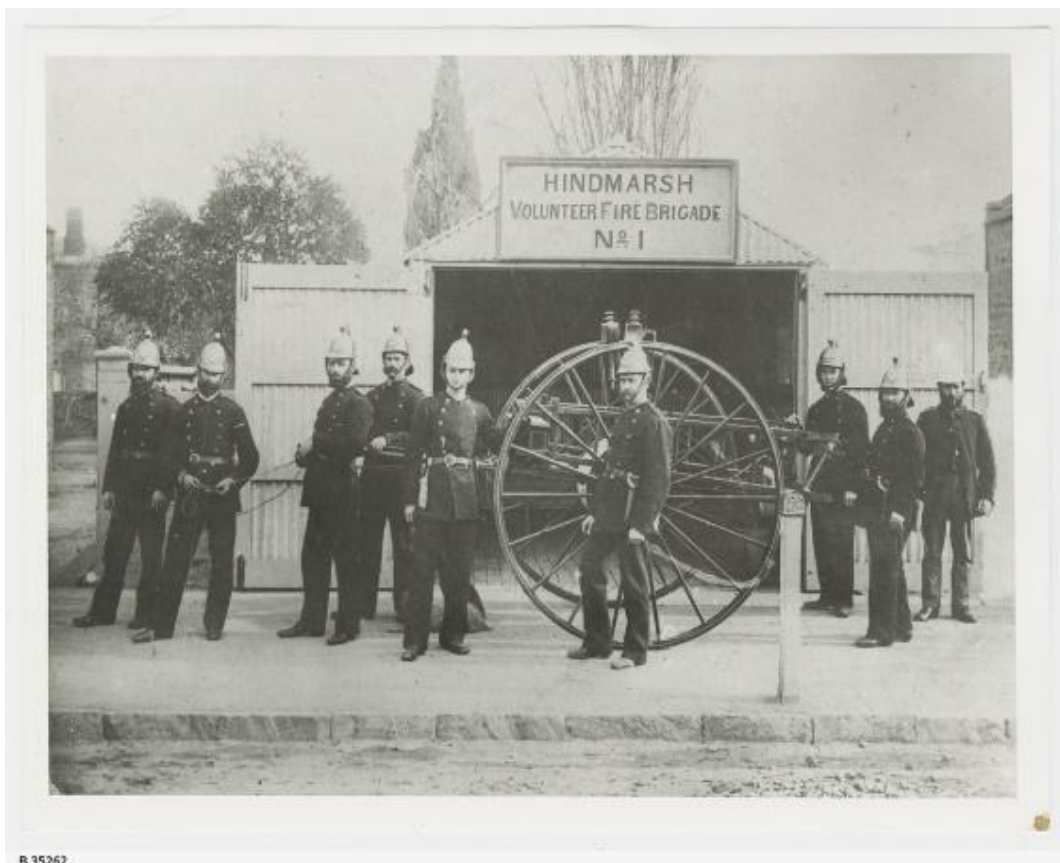
State Library of South Australia - Fire Brigade, Hindmarsh [B 35262], Hindmarsh Volunteer Fire Brigade with a fire hose reel. Approximately 1890. Part of Hindmarsh Collection.
